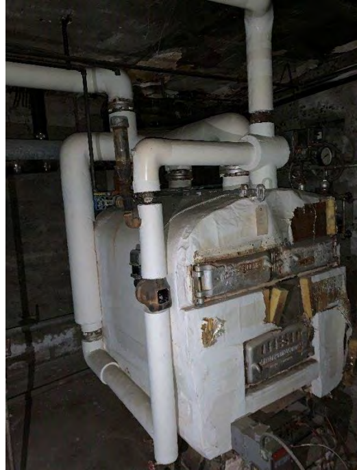
Boiler (fiberglass insulation)
