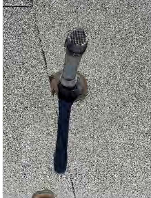
Roofing penetration mastic
