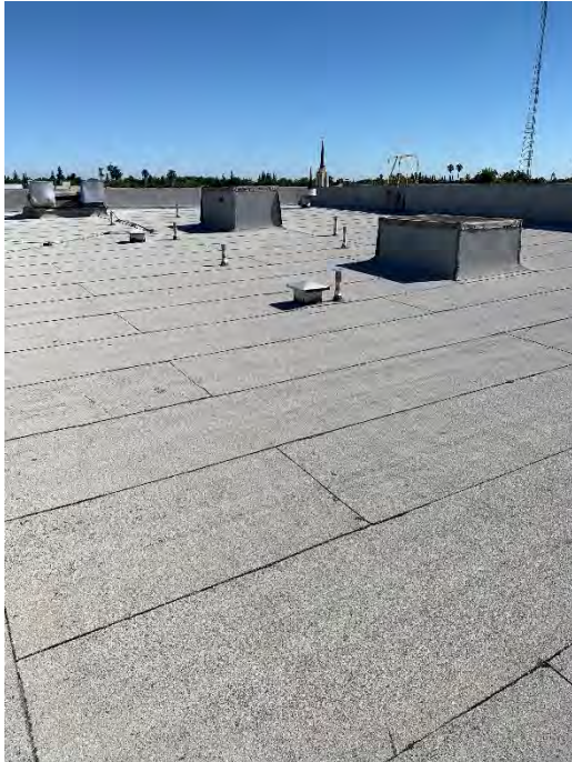
Rolled composition roofing
