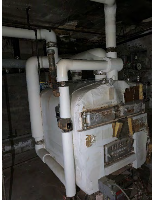
Boiler (fiberglass insulation)
