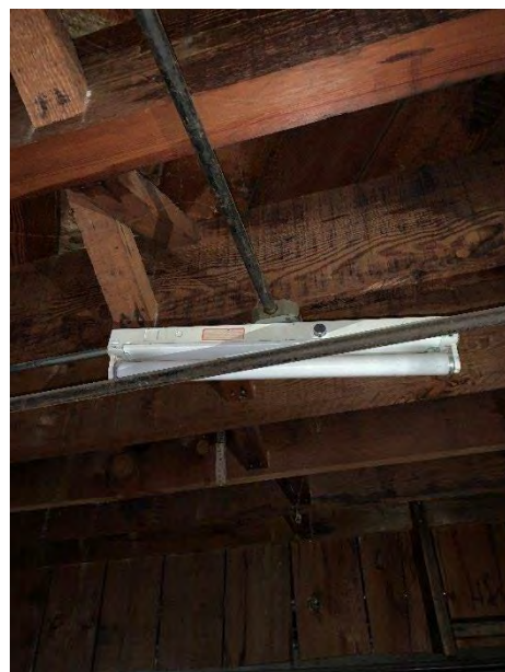
Light ballasts and mercury tubes
