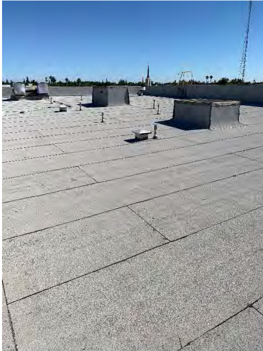
Rolled composition roofing
