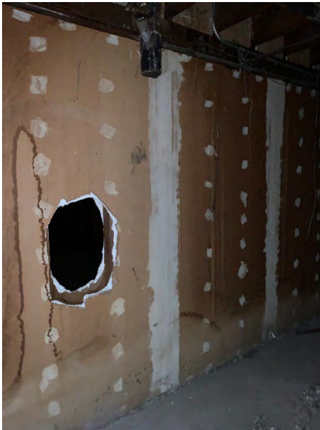
Drywall – Tape and Joint Compound (Basement)
