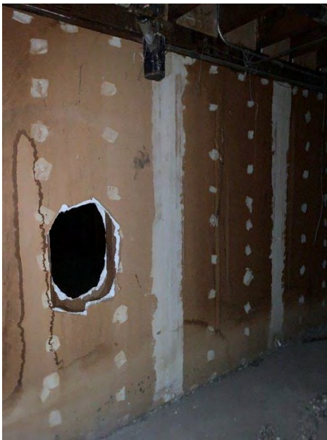
Drywall – Tape and Joint Compound (Basement)
