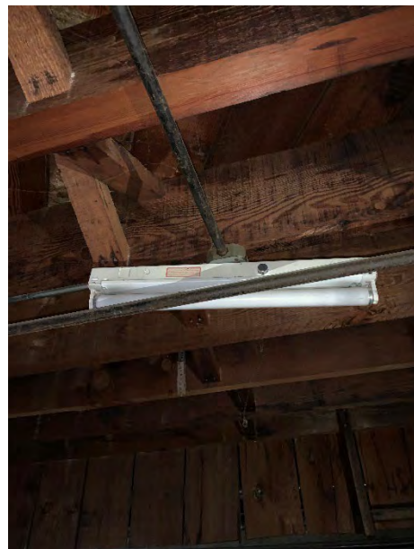
Light ballasts and mercury tubes
