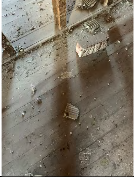
Limited TSI Debris – Third Floor
